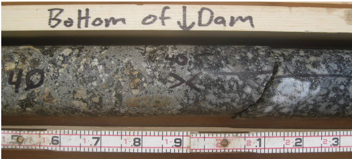
BV-3 from 40.0 to 40.9 feet showing adhered bedrock contact at base of dam
